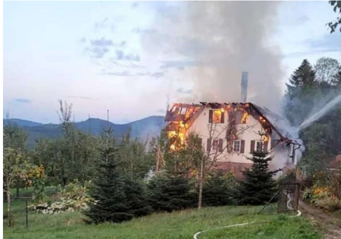
Brand in Oppenau, September 22
